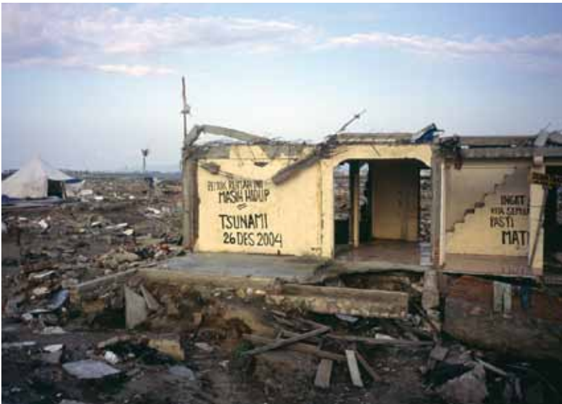
Re-establishing property boundaries and claims is most challenging in post-crisis situation, Banda Aceh, Indonesia. Photo © UN-Habitat / Clarissa Augustinus.
