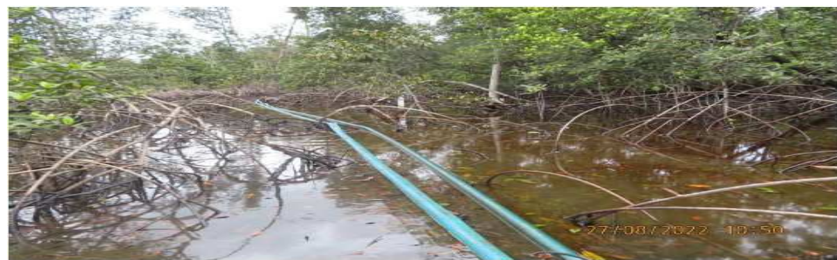
Illegal Siphon Hoses Discovered During Pipelines ROW Surveillance
