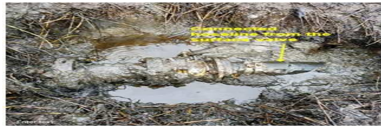
Tapped Point and Illegal Line Connected to the Main Pipeline
