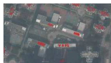
(c) Roof Tops of School
