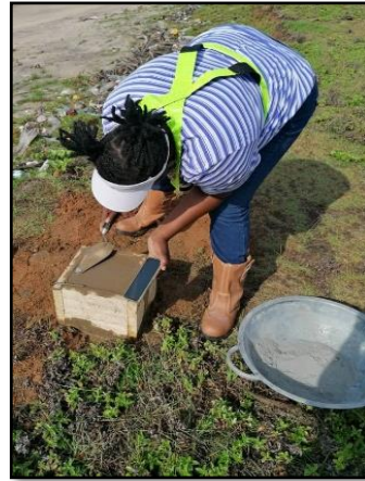
Figure 4: Construction of concrete pillar
