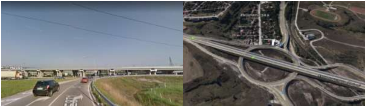
Figure 8: Road junction "Daskalovo"
