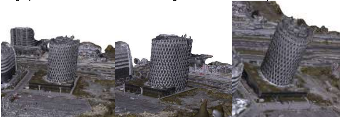
Figure 12: Model of a building on Tsarigradsko Shosse Blvd. obtained as a result of spatial data acquisition with UAS and postprocessing
