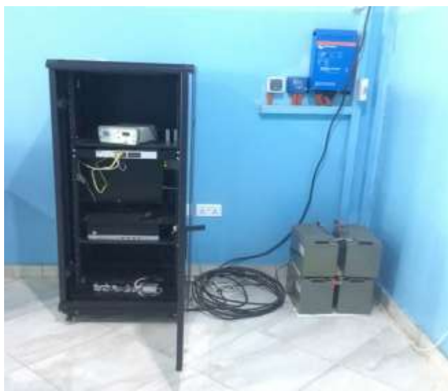
Figure 3: A typical arrangement of LiSAGNet CORS components
