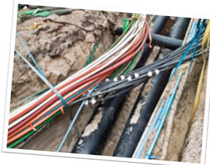
SHIFTING OF EXISTING UNDERGROUND UTILITIES
