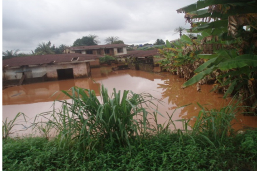
Figure 4: Flooded area by Teachers House in Benin City
