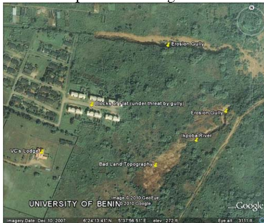
Figure 5(a): Satellite Imagery of University of Benin Erosion Gully Site I
