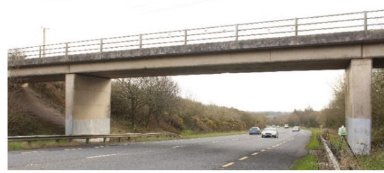
a) Photo of the bridge
