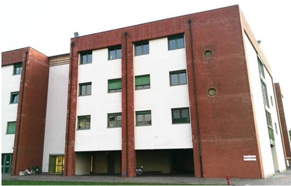
Figure 1. North-East façade of the considered building.
