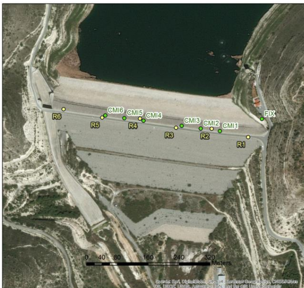
Figure 2: Instrumentation on the dam crest
