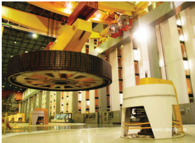
Figure 3 The rotor during its transport
