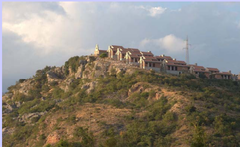
“Village” : illegal settlement without connection to municipal infrastructure for fresh water and sewerage system
