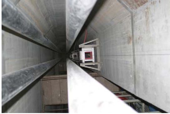
Figure 17: Wire pendulum in pylon head
