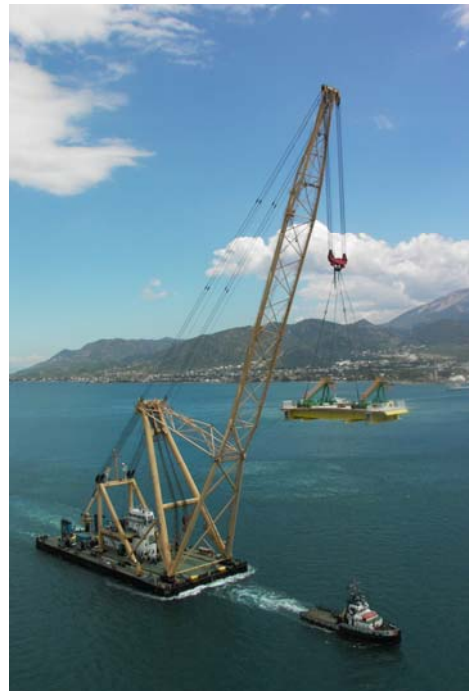
Figure 4: Taklift floating crane
